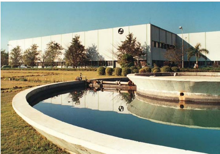
Switchgear Factory, Ahmednagar
