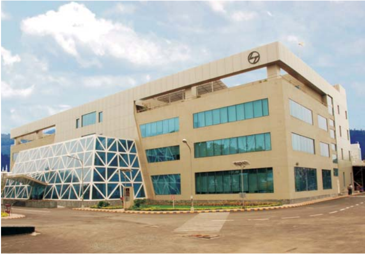
Switchgear Factory, Navi Mumbai
