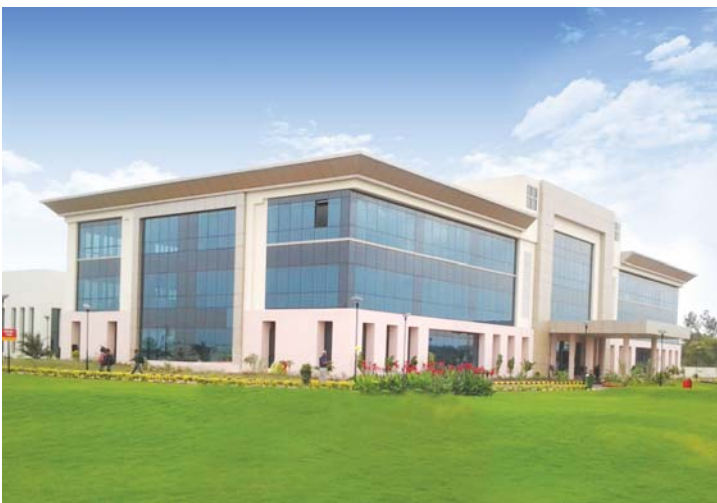
Switchgear Factory, Vadodara
